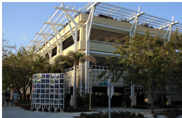
6th Avenue Parking Garage
