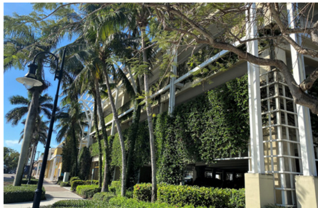
4th Avenue Parking Garage
