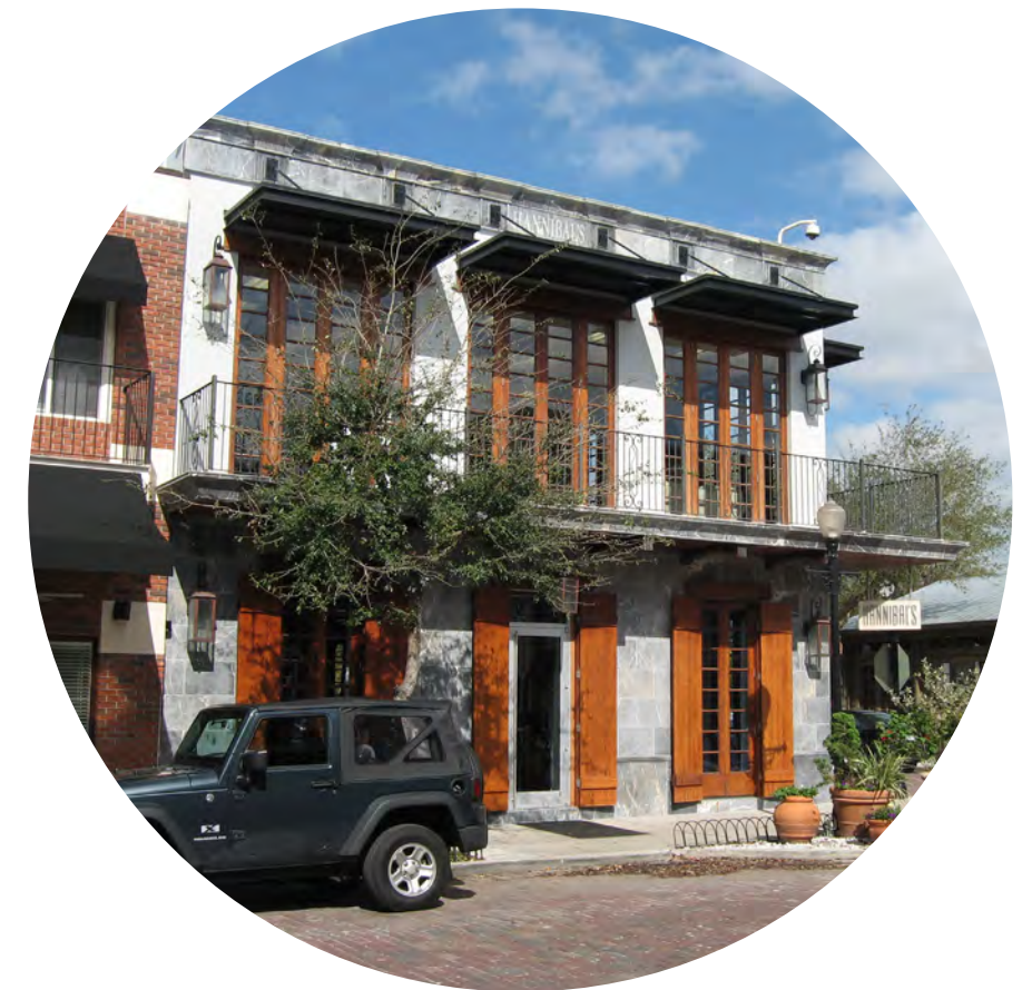
Mixed-Use Building, Winter Park
