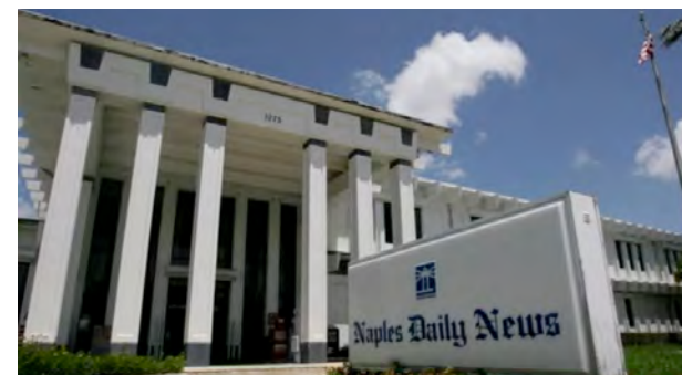
Former entrance of Naples Daily News on Central Avenue.
