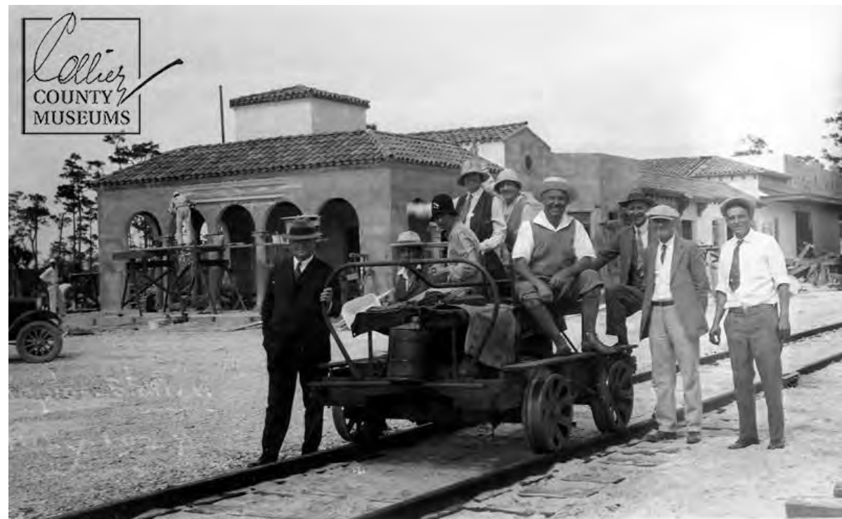
The Railroad Depot Under Construction
