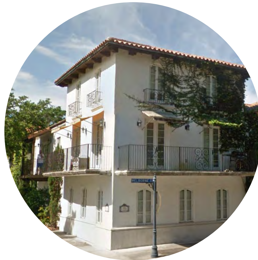
Apartment Liner Building- Winter Park, FL
