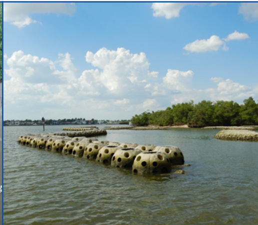
Outer reef balls providing wave attenuation and fish/oyster habitat.
