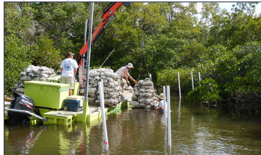
ABOVE: Volunteers placing shell-filled bags at Site 3 to create new reefs near the mouth of Rock Creek adjacent to the Gordon River. BELOW: Garland and Garland Marine Construction donating time and barges to deploy shell bags at Site 3 restoration area.
