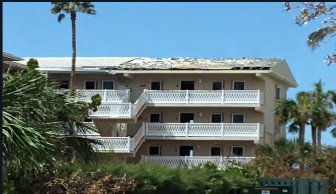
Roof tiles blown off from high winds
