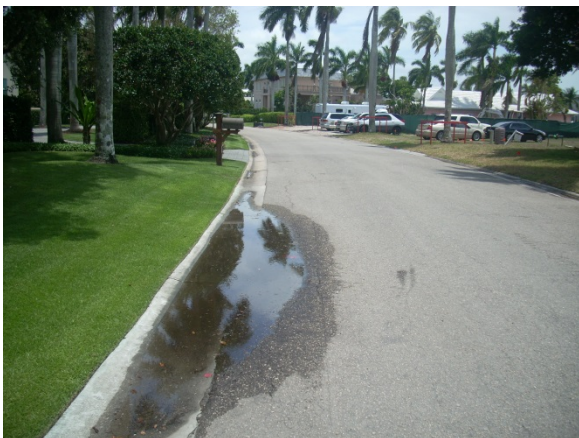
Nelson's Walk – Curb replacement to correct major areas of ponding and coordination during resurfacing with four Single Family New Homes under construction
