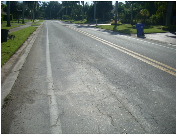
Orchid Drive – Resurfacing along with leveling coat to correct wheel rutting and add structural strenght to the roadway
