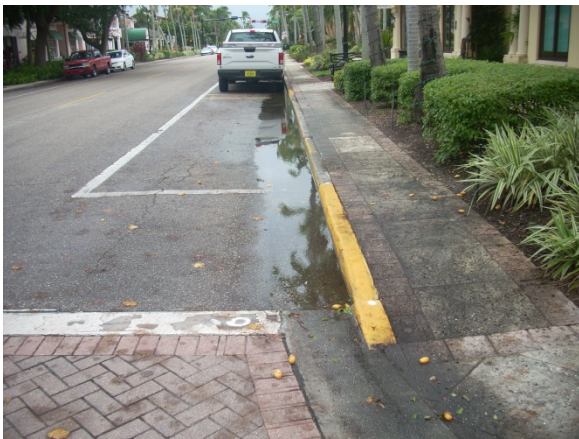
5 th Avenue South – Curb replacement to correct major areas of ponding and repair damage from tree root upheaval. Biobarrier was installed to prevent future root damage
