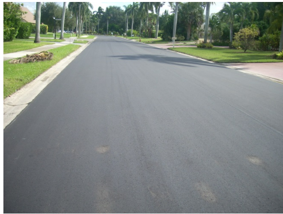
Orchid Drive – Resurfacing along with leveling coat to correct wheel rutting and add structural strenght to the roadway
