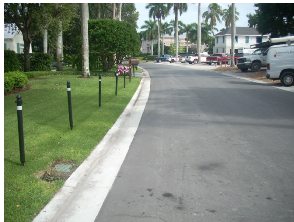
Nelson's Walk – Curb replacement to correct major areas of ponding and coordination during resurfacing with four Single Family New Homes under construction
