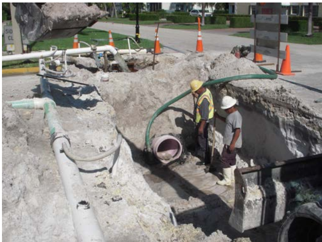
Stormwater inlet & pipe repair 7 th Ave S & 3 rd St South prior to Streets Division resurfacing
