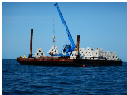
Artificial Reef module deployment (April 2016)
