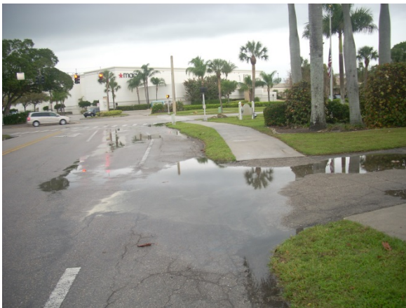
10 th Street North – Resurfacing along with swale installation and leveling coat to correct areas of roadway ponding
