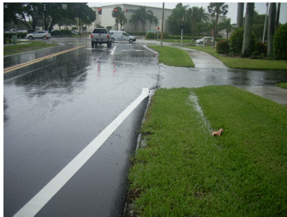
10 th Street North – Resurfacing along with swale installation and leveling coat to correct areas of roadway ponding
