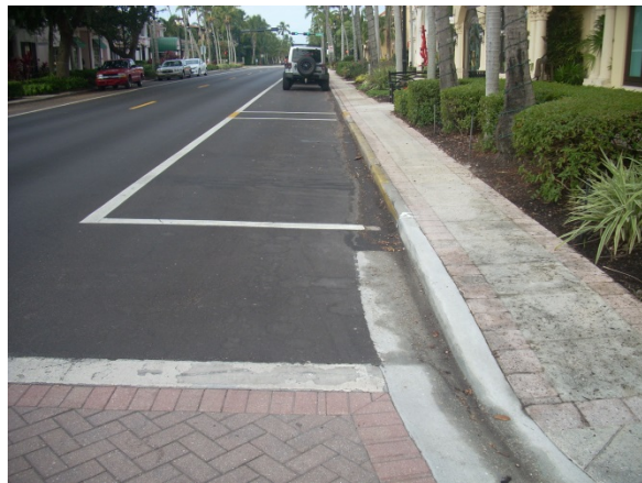
5 th Avenue South – Curb replacement to correct major areas of ponding and repair damage from tree root upheaval. Biobarrier was installed to prevent future root damage
