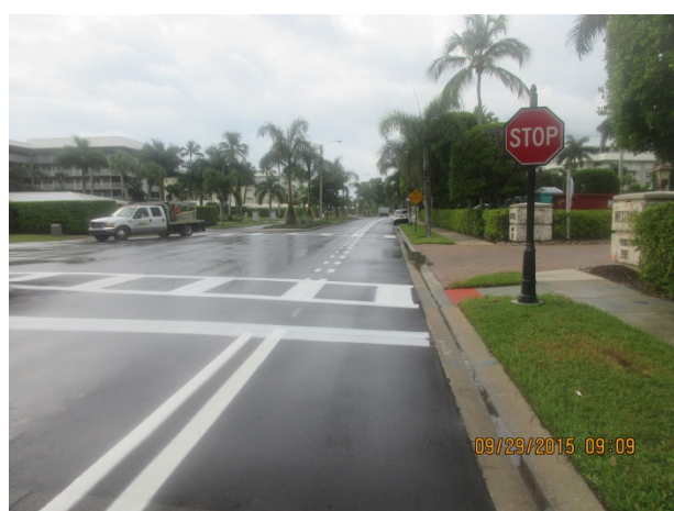
Gulf Shore Blvd North & Harbour Drive - Crosswalk improvements including ADA compliance and the new 6" buffered bike lane line for safety.
