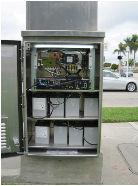
FDOT provided the city with 20 new traffic signal cabinets and battery backups for intersections on US41.
