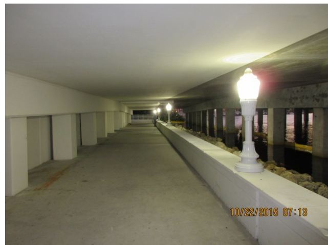
Gordon river underpass improvements – New guardrail, paint, lighting, replacement of ramps to meet ADA standards, under mounted gutter for drainage, signage and new cameras added by the City for safety
