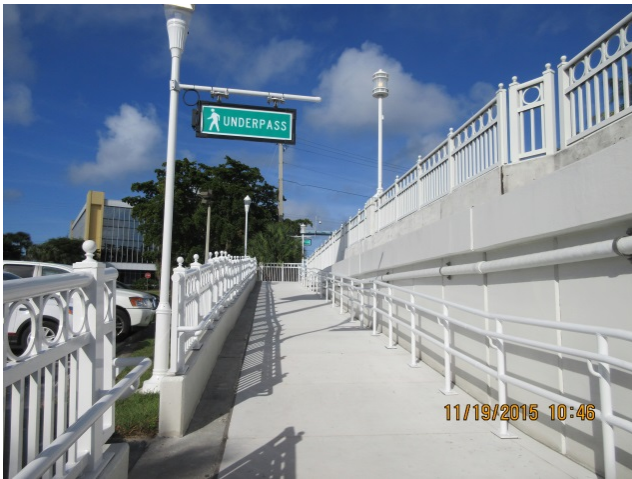
Gordon river underpass improvements – New guardrail, paint, lighting, replacement of ramps to meet ADA standards, under mounted gutter for drainage, signage and new cameras added by the City for safety
