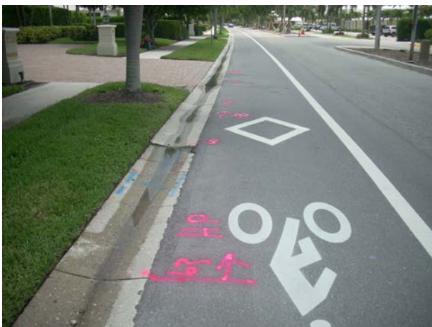
Gulf Shore Blvd North & Harbour Drive - Crosswalk improvements including ADA compliance and the new 6" buffered bike lane line for safety.
