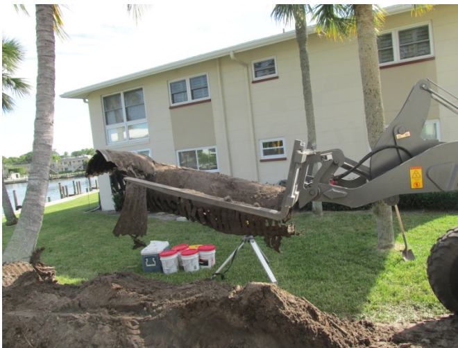
Metal pipe replacement at 1550 Gulf Shore Blvd N
