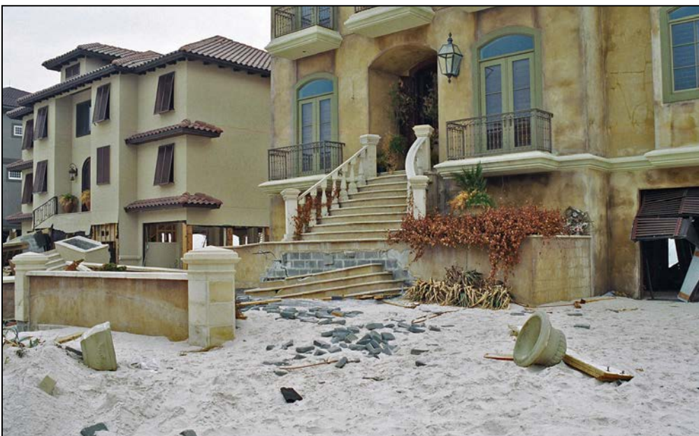
Figure 3: Massive stairs attached to an elevated coastal home, which act as an obstruction
