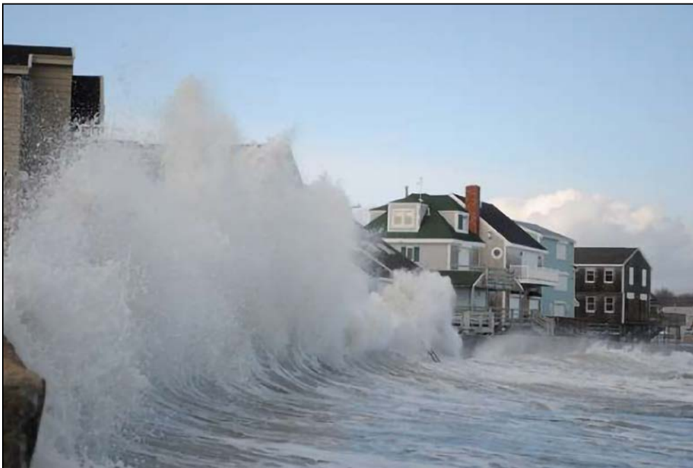
Figure 24: Wave runup and overtopping at an erosion control structure
