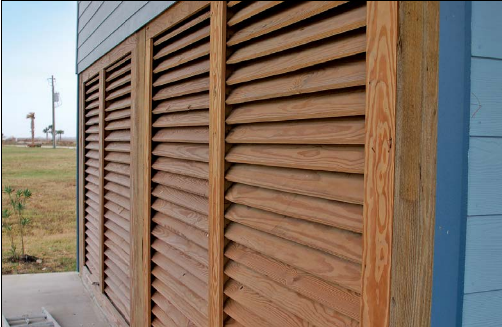
Figure 5: Compliant, fixed, wood louvers installed between pilings
